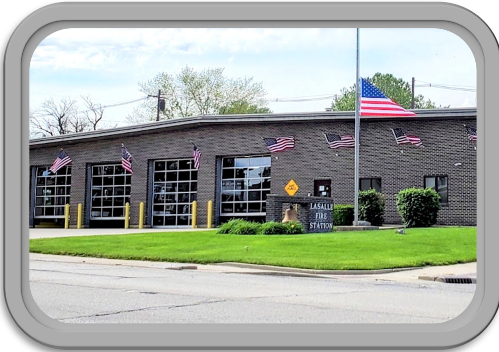
LASALLE FIRE STATION
